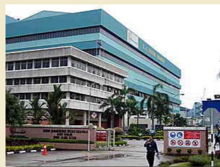
RISKWISE™ application at TNB's Pasir Gudang power station in Malaysia
