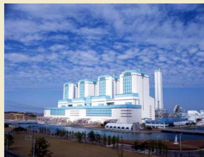
Application to boilers, steam turbine and balance of plant at Korea East-West Power Company's Danjing supercritical plant
